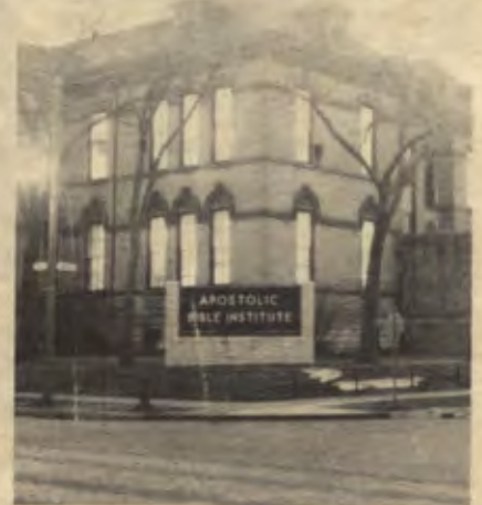
School at 745 Grand Avenue
